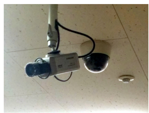
One of the new cameras to be installed in dorm rooms.
